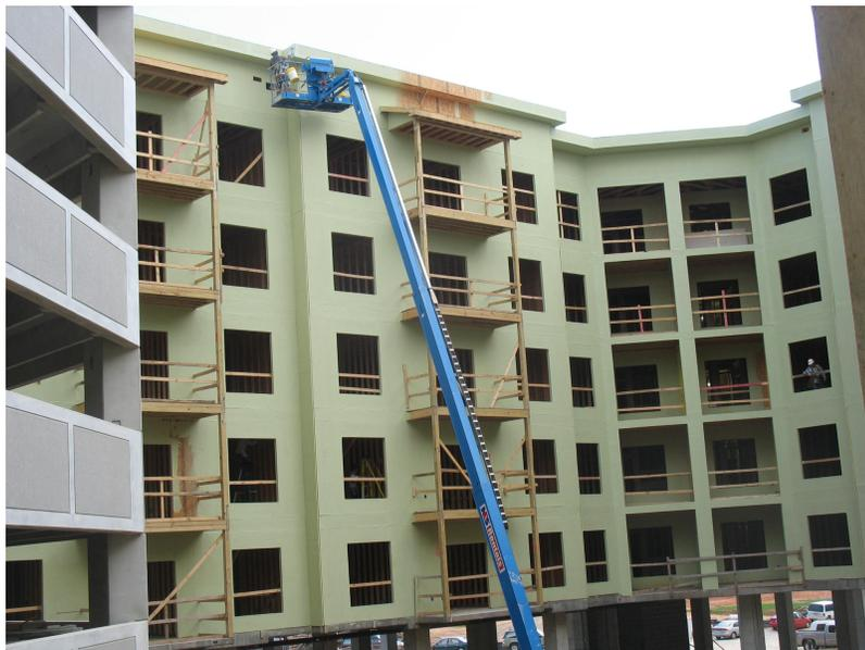
Application of liquid weather resistive barrier to wood framed building. Liquid weather barriers offer greater protection and are less susceptible to weather damage before the wall cladding is applied than their paper and fibre counterparts.
